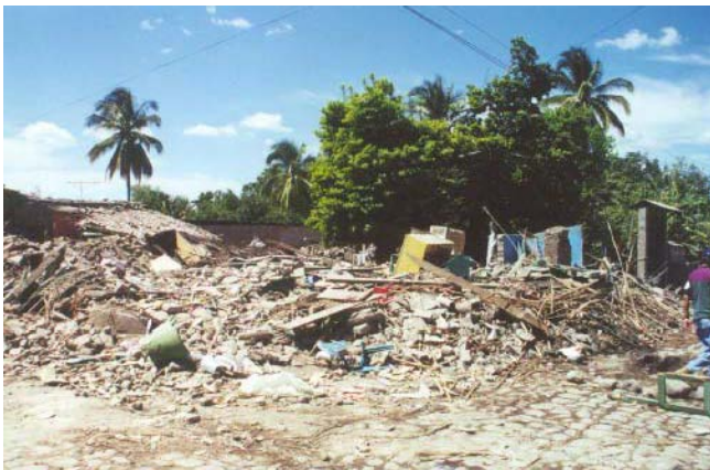
Figure 1.1 Damage of brick masonry building in Bhuj Earthquake (2001)
